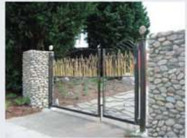
McConnell Ave Gateway along Ballona Creek
