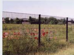
Double wire fence
